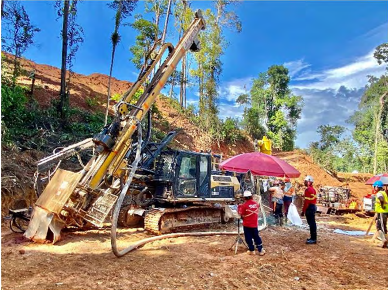
Figure 10.4: Reverse Circulation Rig (compressor and booster not shown)
